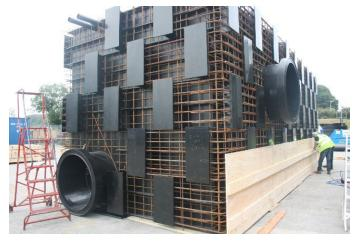
Optional timber shuttering can be factory fitted to accept the site installed insitu concrete poured surround.
