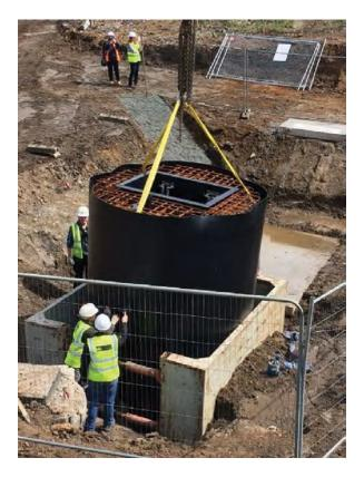
Rising mains, guide rails, valves and if applicable flow meters are factory fitted.
